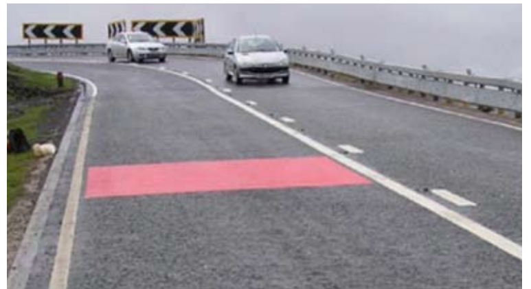
Figure 22 Red paint on pavement warns for caution in a dangerous curve (from EuroRAP's Barrier to Change: Designing Safe Roads for Motorcyclists). Photo – Cheshire County Council, UK
