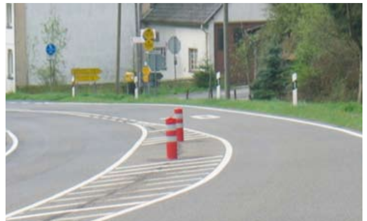
Figure 39 Flexible bollard in a curve versus a rigid sign post (Germany). Photo – Biker Union E.V.
