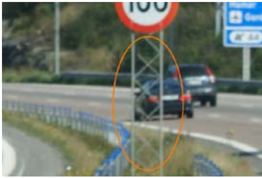
Figure 40 Breakaway lattice on a 100 km/h sign (Norway). Photo – J. Baron
