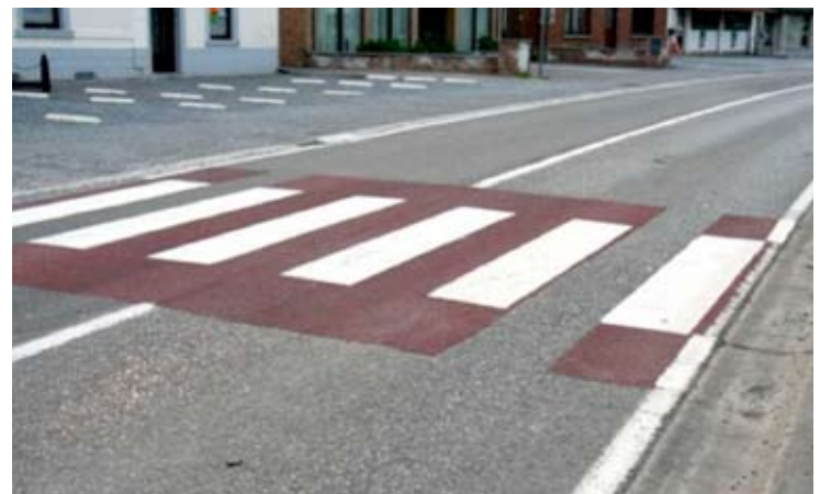
Figure 28 In recognition of the effects of slick pavement markings, the authorities specify a 0.5 meter “gap” for motorcyclists and bicycles to pass through in this crosswalk (Belgium). Photo – Benoit Dupriez
