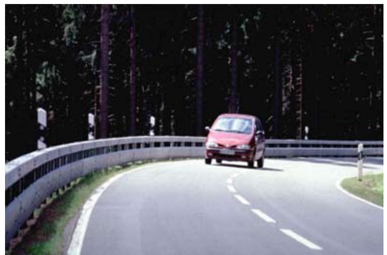
Figure 8 Box Beam (Germany) Photo – Uwe Ellmers
