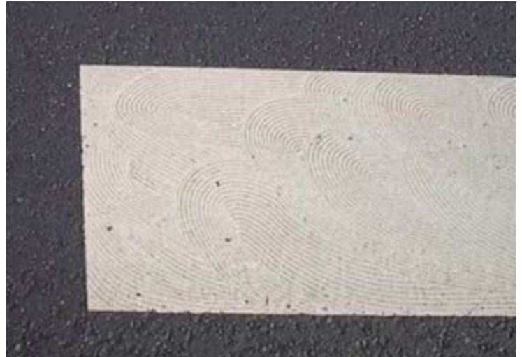
Figure 27 Pavement marking with a “textured” surface for skid-resistance achieved by “trowling” heated thermo (Belgium) Photo – Benoit Dupriez
