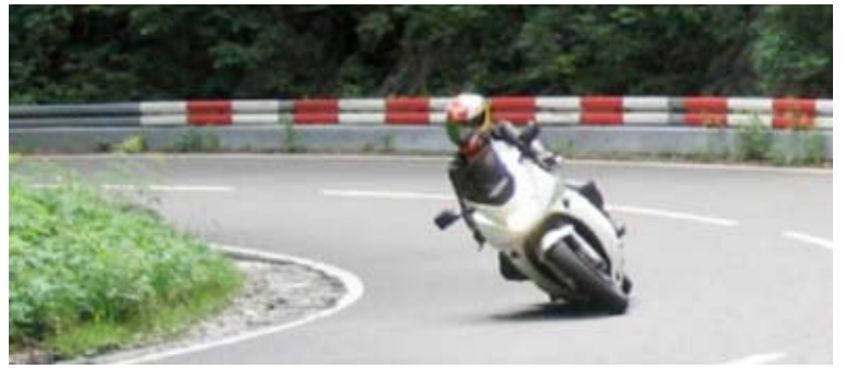
Figure 20 Reflective white and red sheeting is applied to the top of motorcycle guardrail in a curve. Image from EuroRAP's Barrier to Change: Designing Safe Roads for Motorcyclists. Photo – ADAC, Germany
